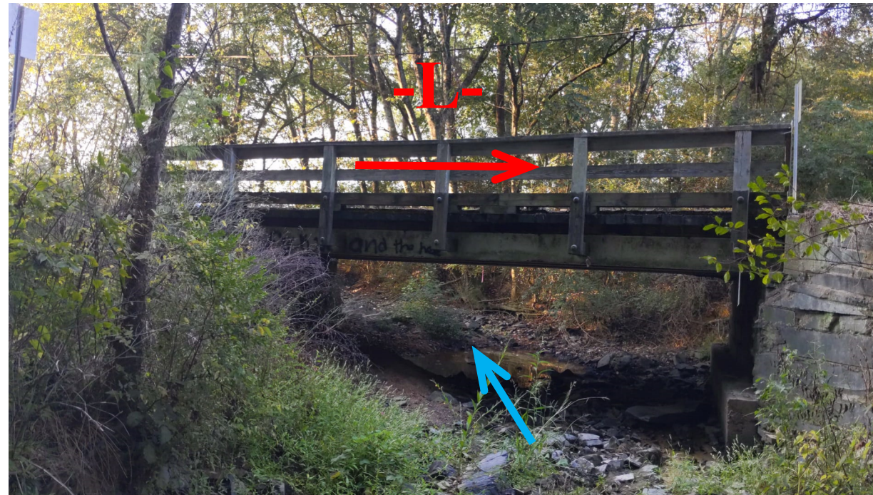
Looking North from South Side of Bridge
